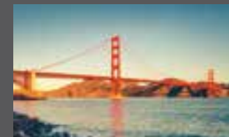
Golden Gate Bridge
